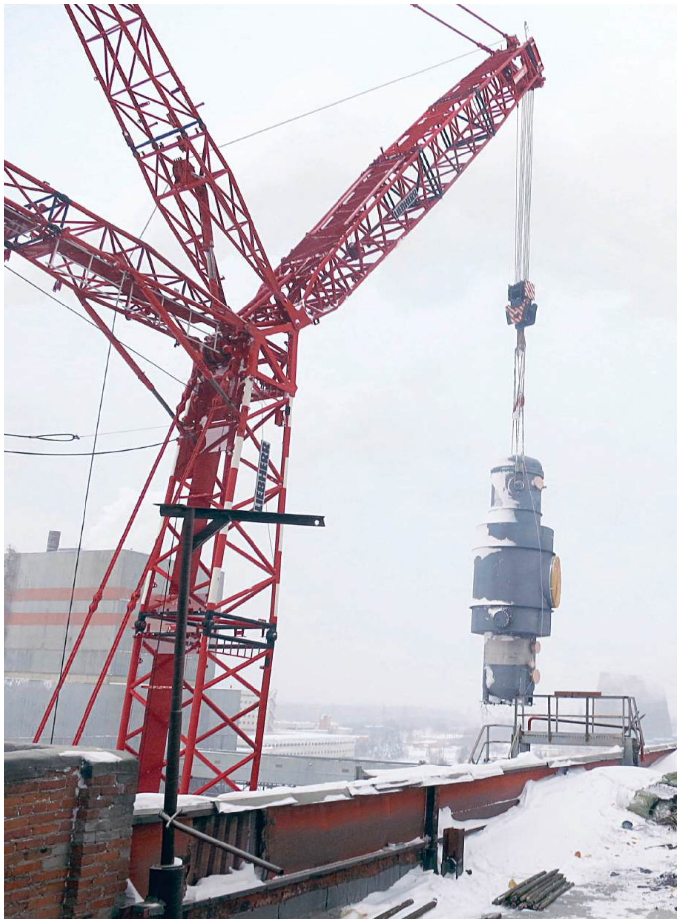
Pulp mill, Ust-Ilimsk city, Irkutsk region. Installation of evaporation station equipment.
