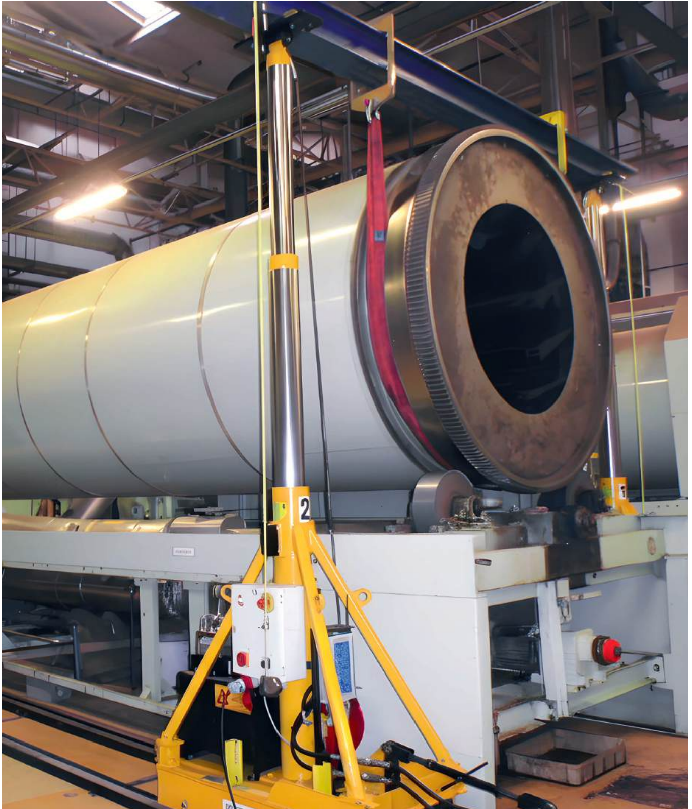
Tobacco factory, Samarkand city. Installation and assembly of a 17-ton drum.
